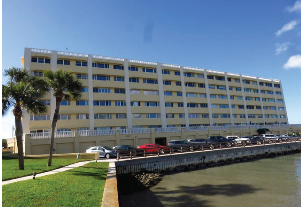
3 Rear of House
