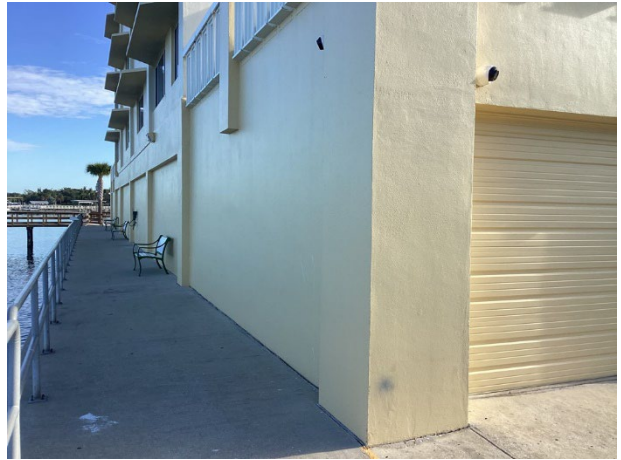
Stucco wall finishes
