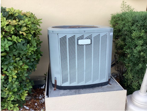
Split system condensing unit for the lobby
