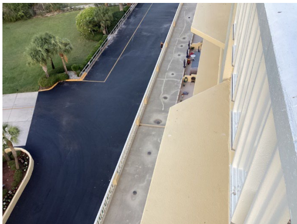
Thermoplastic lower roof overview
