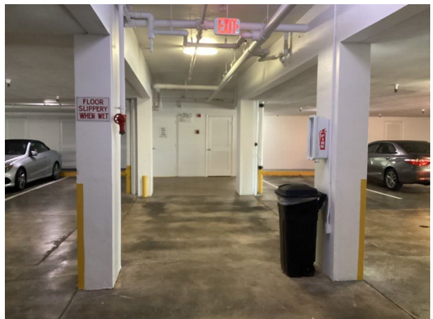
On-grade garage columns overview
