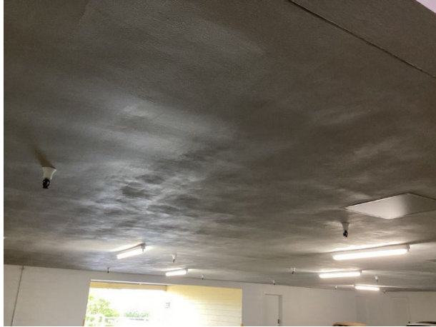
Fire suppression system
