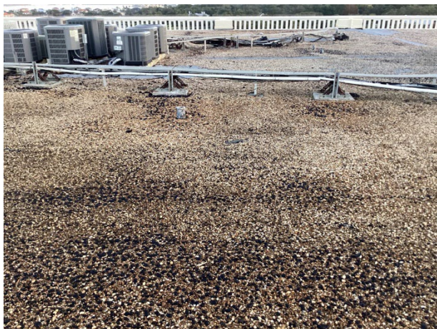
Built-up upper roof overview
