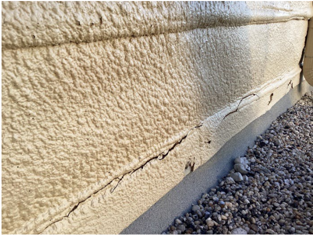
Stucco cracks
