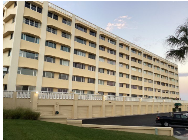
Rear elevation of building
