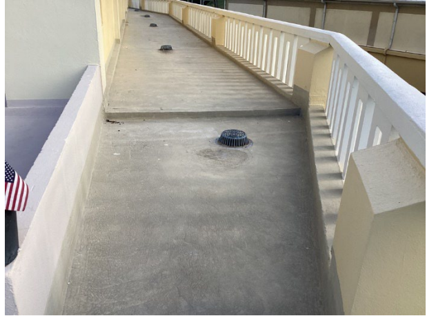
Thermoplastic lower roof overview
