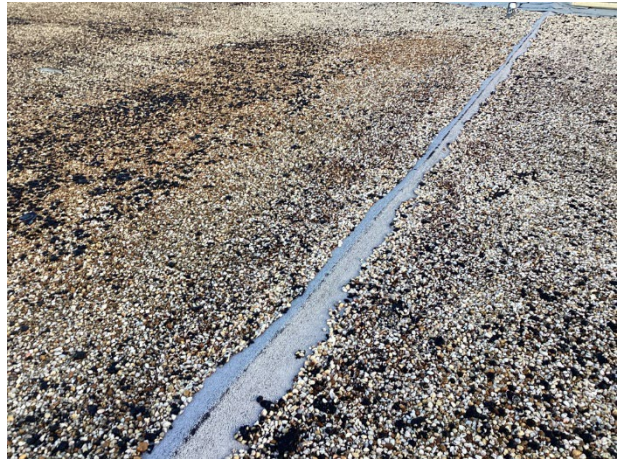
Ridging at the upper roof
