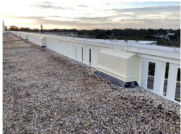
Concrete safety railings at the roof
