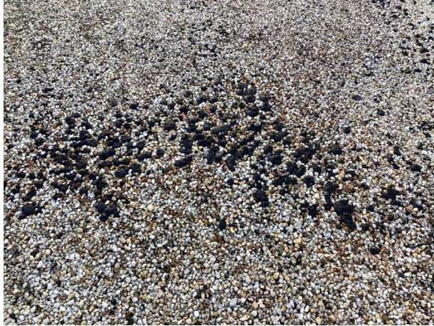
Ballast encapsulation at the upper roof
