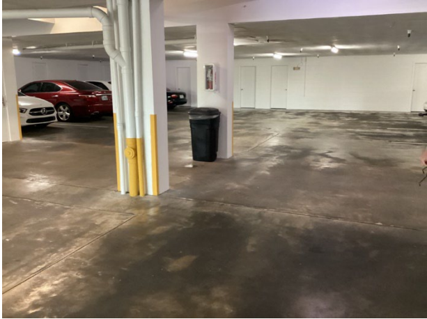
On-grade garage floor overview
