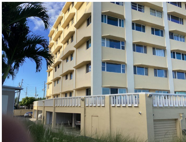
Side elevation of building
