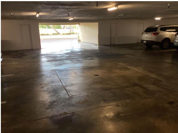
On-grade garage floor overview
