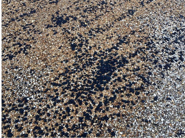
Ballast encapsulation at the upper roof
