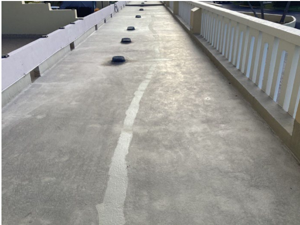
Thermoplastic lower roof overview
