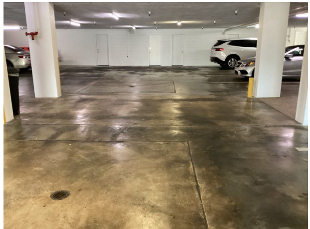
On-grade garage floor overview
