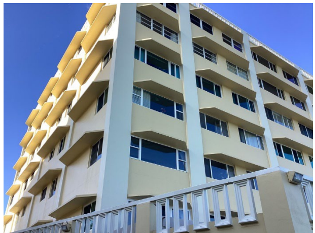
Stucco wall finishes
