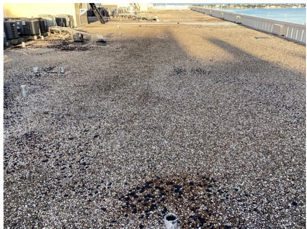
Built-up roof overview
