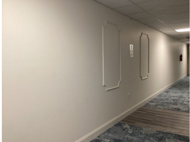
Paint finishes at the hallways
