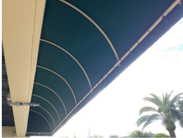
Awning underside overview
