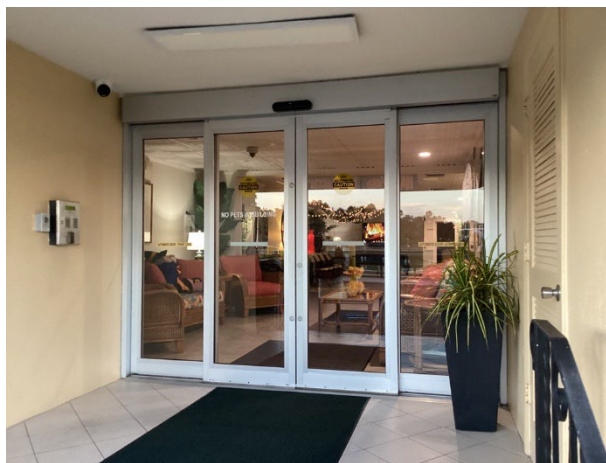
Common windows and doors at the main lobby entrance
