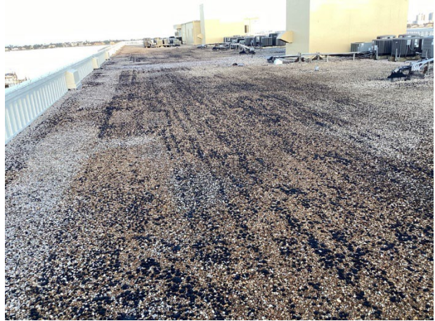
Built-up upper roof overview
