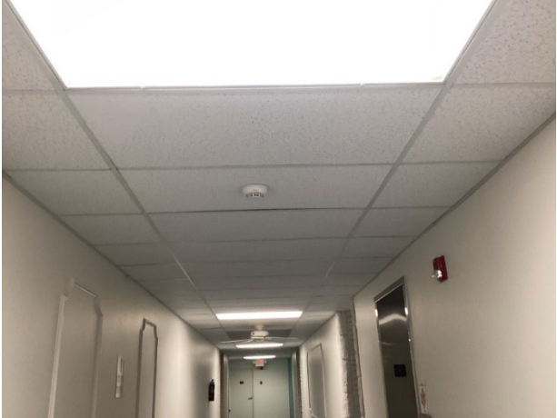
Acoustical ceiling tiles at the hallways
