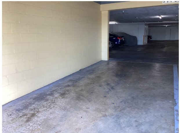
Paint finishes at the garage
