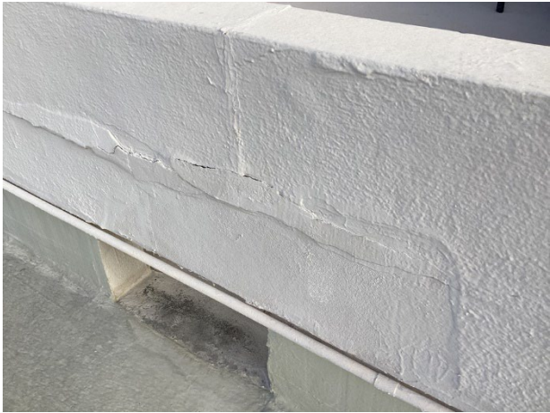
Stucco cracks
