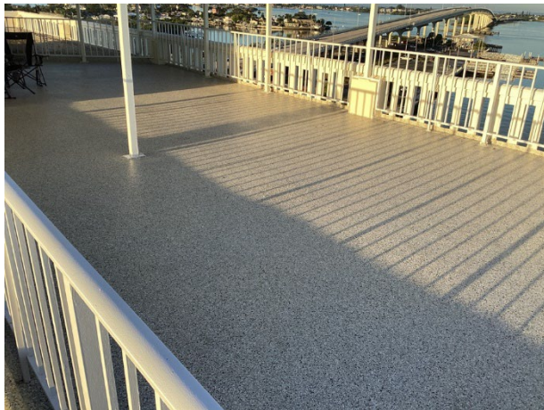
Rooftop balcony overview
