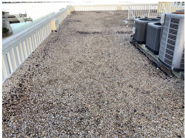
Built-up upper roof overview
