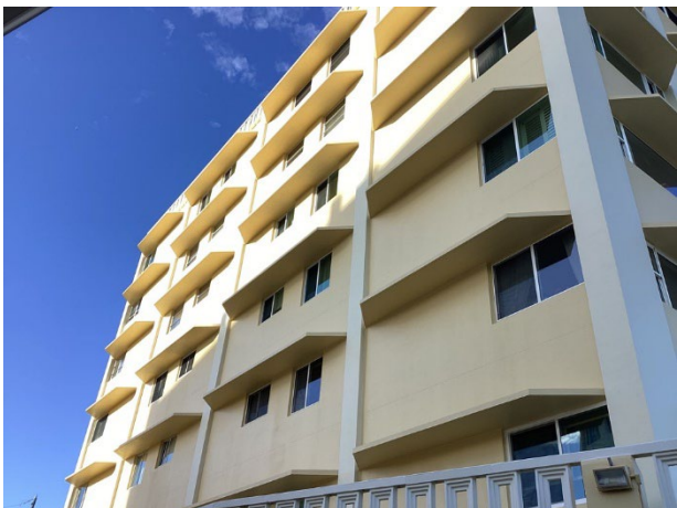
Stucco wall finishes
