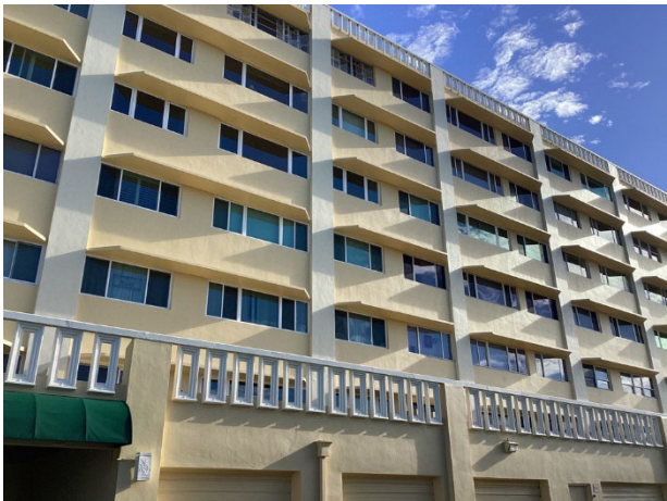
Stucco wall finishes and concrete railing finishes
